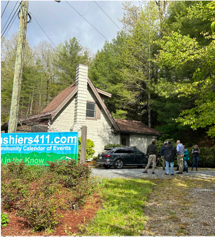
Cashiers Area Chamber of Commerce and site access facing US 64.
